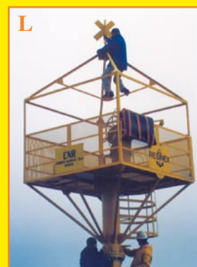
L: when platform is ready, details are assembled
