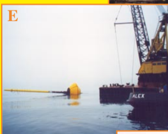
E: float, metallic part and sinker are carried by the pontoon to the laying place
