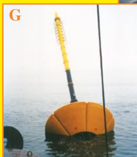
G: the sinker is lowered
