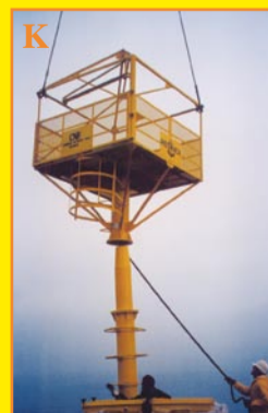
K: the platform (6,25 sq.mt) is easily positioned on the upper part of the pipe
