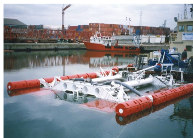
The complex shallow water trenching machine.
