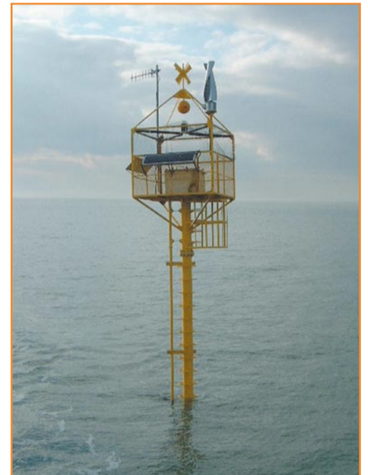
The beacon operating at Shivering Sands
